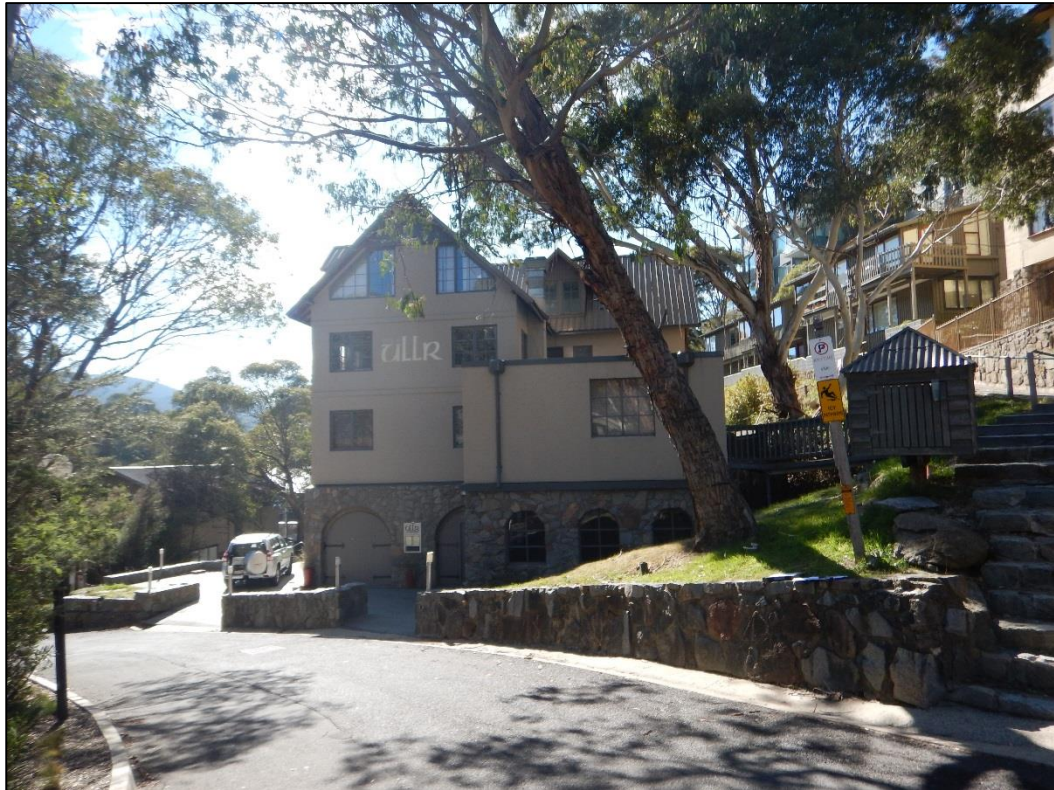
Plate 1: Western elevation of House of Ullr
